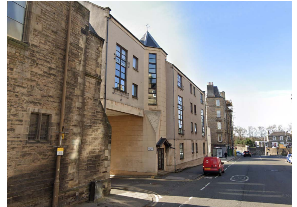
2. View of neighbouring residential buildings on Rodney Place
